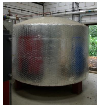
'Large' accumulator working with a 250kW boiler to heat a former stately home (or 'schloss')
