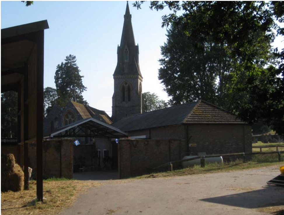
Fig. 2: Proposed site of the heating plant (horse barn)
