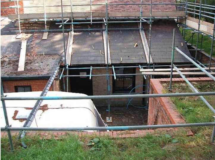
Fig. 4: Wood chips bunker
