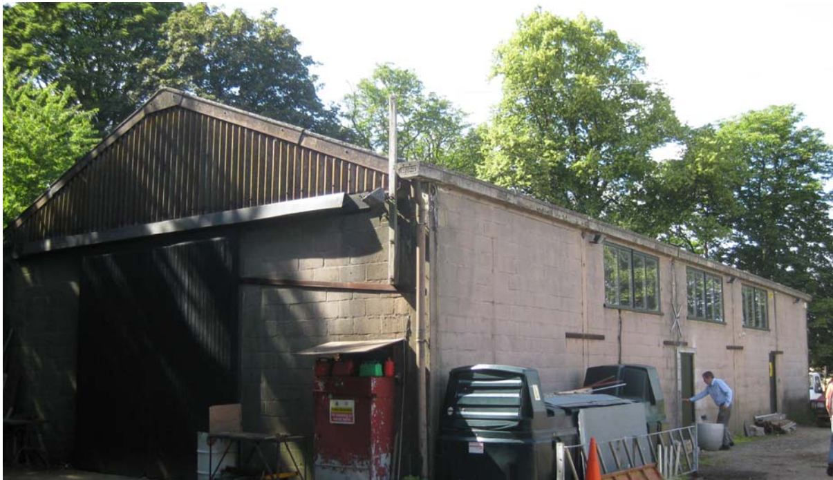
Fig. 2: Existing fuel storage
