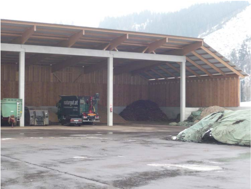
Fig. 3: Example of fuel storage in Austria
