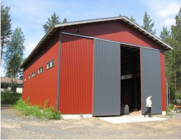
Figure 2: A 0.7 MW heating plant. Photo: Jyrki Raitila, VTT.
