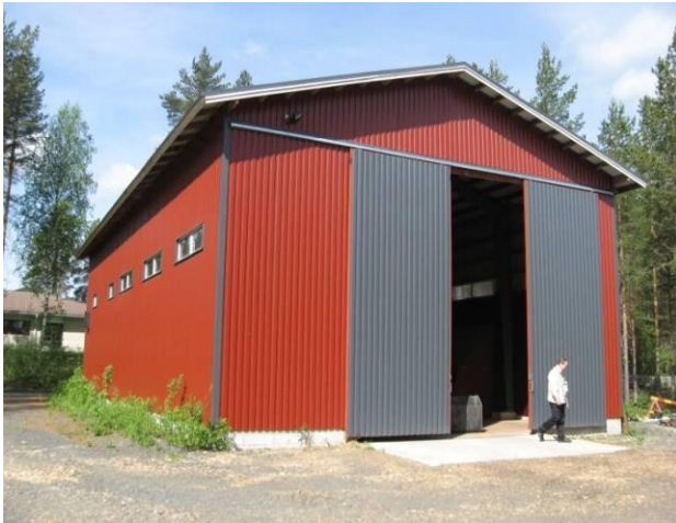
Figure 3: A 0.7 MW heating plant. Photo: Jyrki Raitila, VTT.
