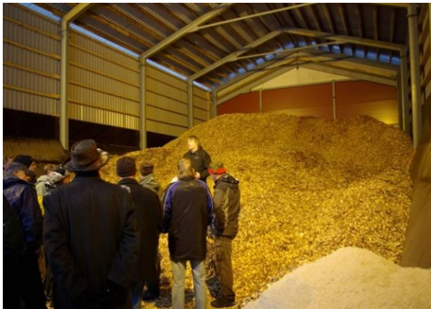
Figure 4: A chip store (boiler right behind the wall). Photo: Jyrki Raitila, VTT.
